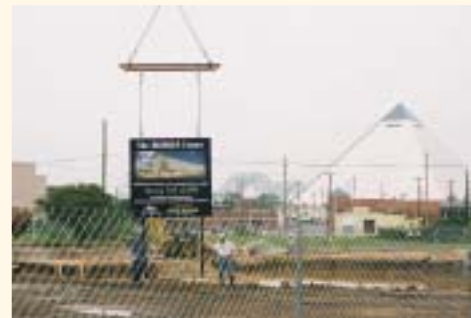
Bridges, Inc. headquarters gets underway in Uptown.
